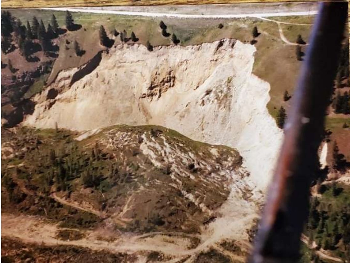
Photo – 1984 slope failure
