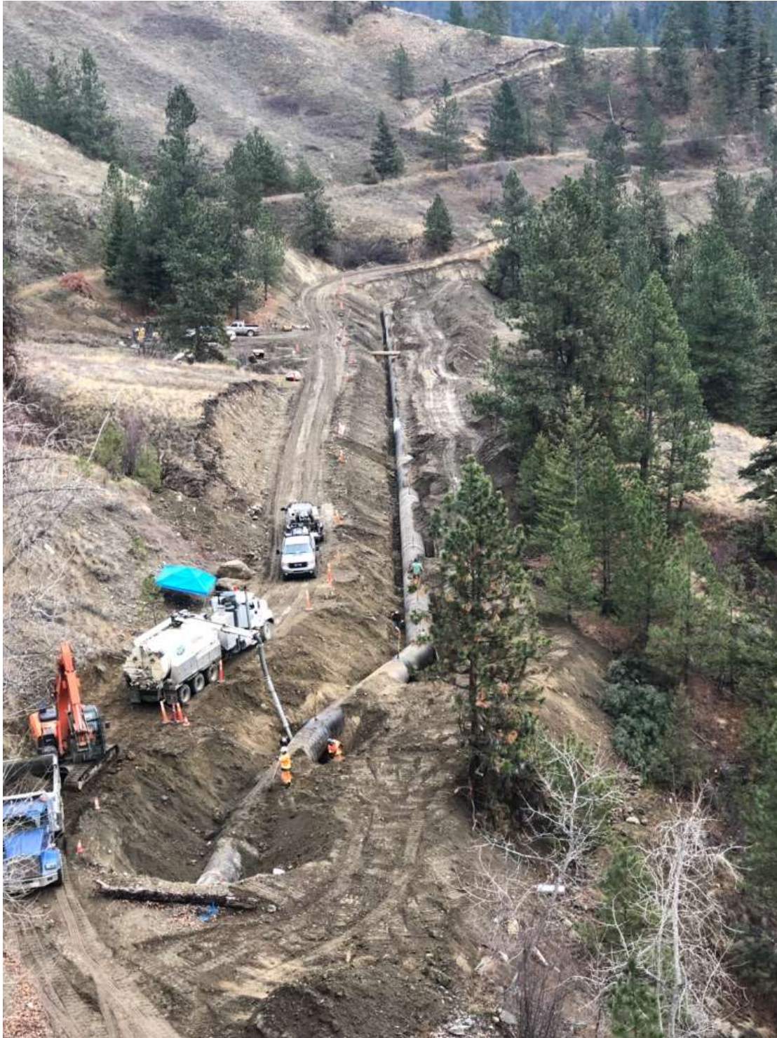
2018 Photo – Relieving upstream slope pressure on BMID 1500mm diameter transmission main
